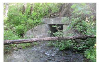
Figure 1: Existing Prestile Brook Culvert
